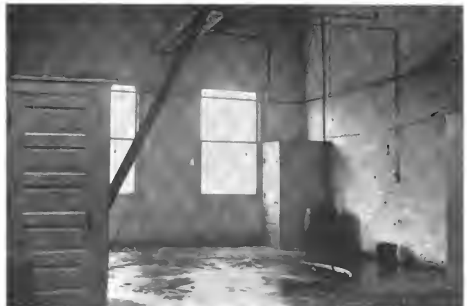
WASH RACK WITH TURNTABLE IN ATWOOD GARAGE.
